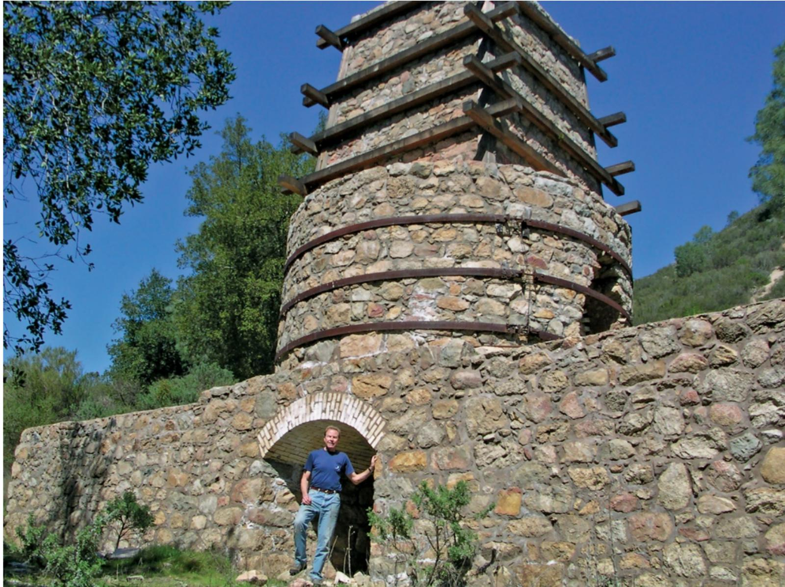
This kiln was built circa 1860 for use in processing limestone rock for use in cement and mortar. The rock pieces were “cooked” at high heat for 24 hours.
