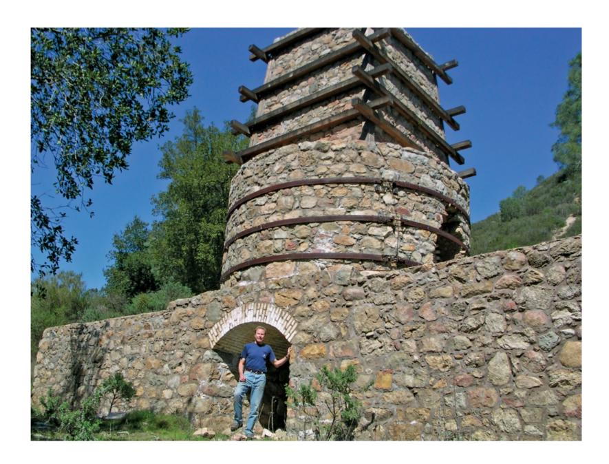
This kiln was built circa 1860 for use in processing limestone rock for use in cement and mortar. The rock pieces were "cooked" at high heat for 24 hours.
