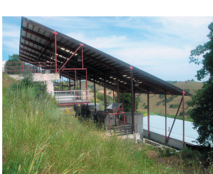
Calera's gravity flow winery pictured here was a necessity since there was no electricity when the winery began operations years ago. Now it is a natural energy saver.
